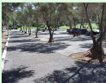
The above parking lot incorporates pervious pavement and depressed landscaping islands.
