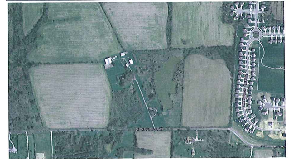
Central Aerial View September 10, 2009
